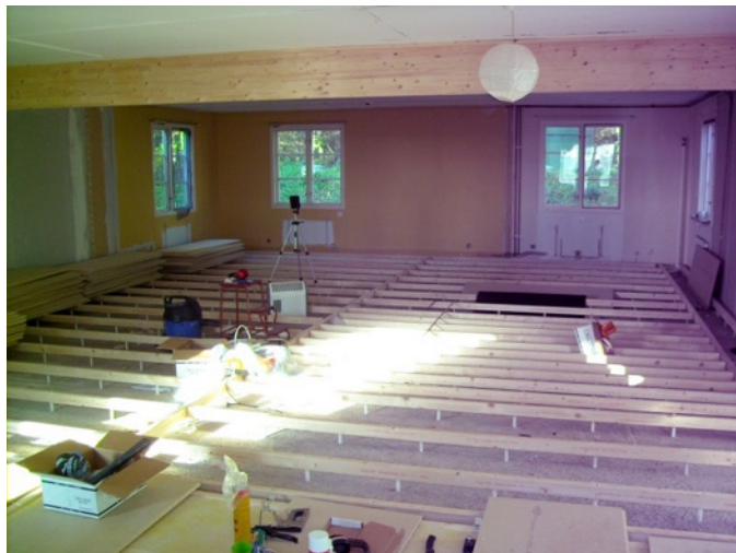
Renovation of the floor in the Dhamma hall
